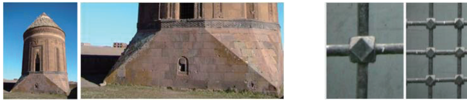
Fig. 7: Cuboctahedron on kumbets and iron window grills
