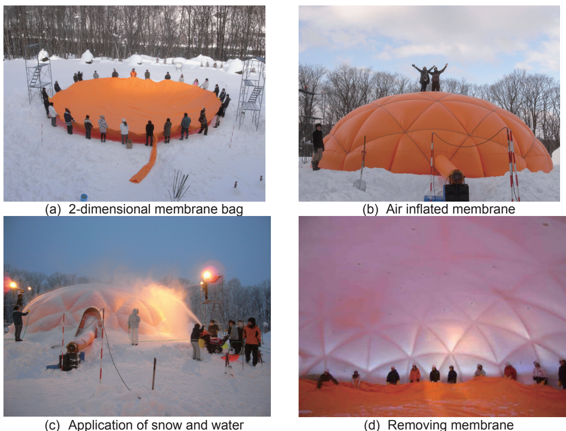
Fig. 2: Construction sequences of 15m ice dome* constructed by students of Tokai University [2]
