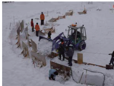
(2) Putting snow and pouring water
