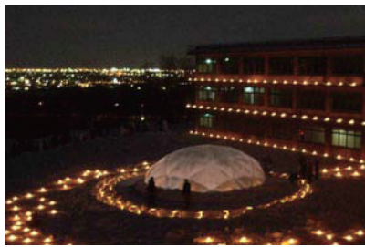
(a) IPP2009 10m Ice dome* (base diameter=8.6m, height=3.0m)
