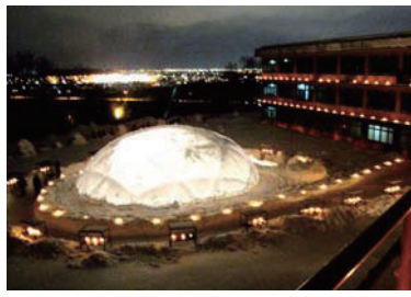
(b) IPP2010 15m Ice dome* (base diameter=12.6m, height=5.0m)
