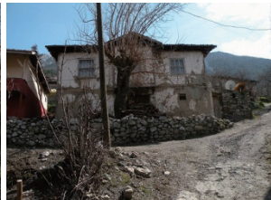
Fig. 22: House with characteristic facade
