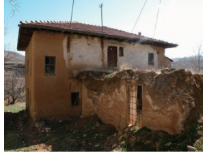
Fig. 33: House with collapsed wooden upstairs in front.
