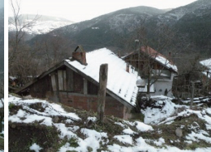
Fig. 13: Masonry walls used in downstairs
