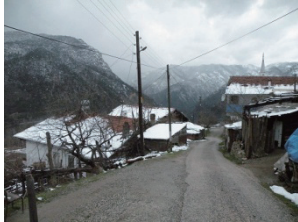
Fig. 10: Downslope road in settlement
