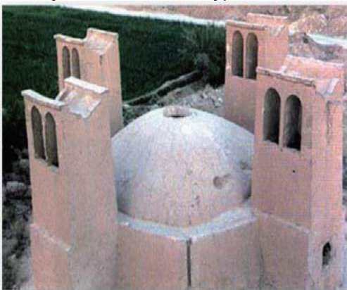
Dowlatabad reservoir with four Kermani deflector in Dowlatabad Garden, Yazd
