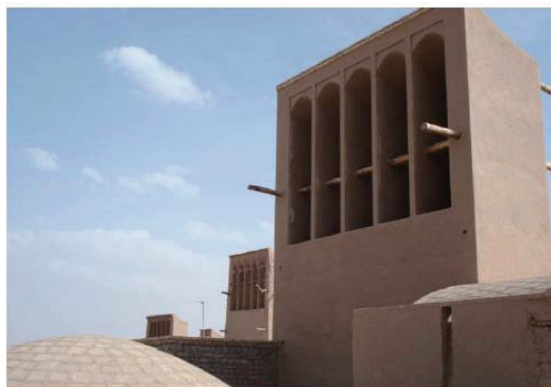
a reservoir with two storage and seven Yazdi deflector in Hossein Abad, near Yazd
