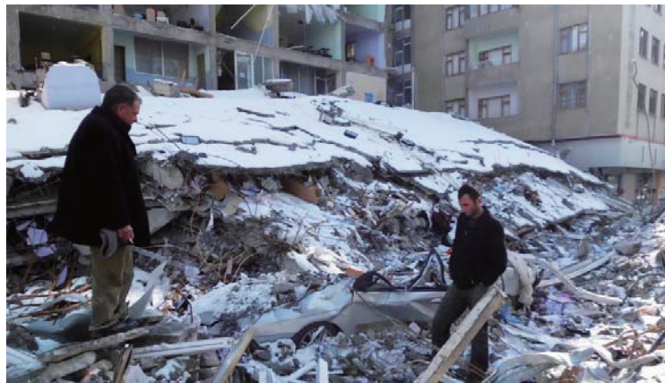
Fig.4: A Photo from 2nd Earthquake
