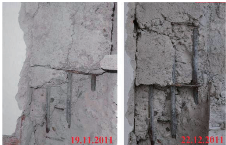
Fig. 5: Increased Damages due to 3rd Earthquake
