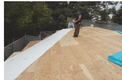
Fig. 7: Full scale drawing placed on roofboards
