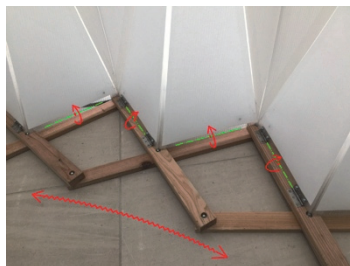
Fig. 6: Joint of folded plate and sill
