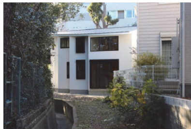
Fig. 10: Appearance from the east side
