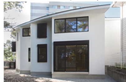
Fig. 11: Appearance of the east side
