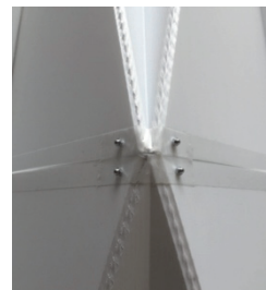
Fig. 7: Reinforcement at vertex
