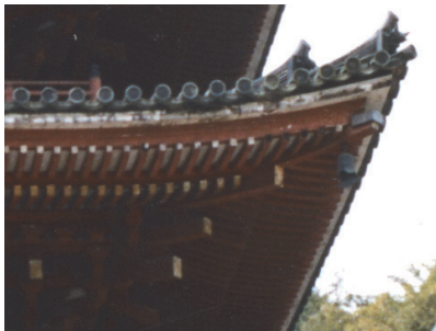
Fig. 3: Myououin, Eaves Rafters
