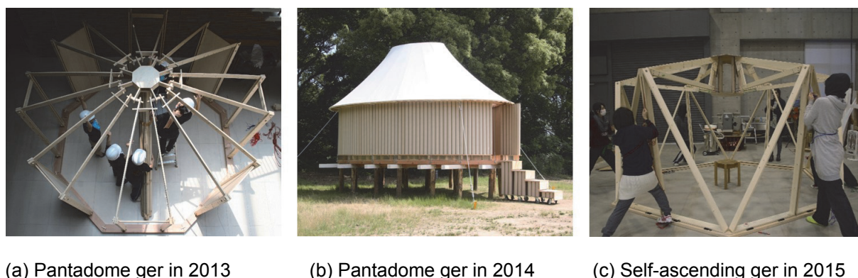
Fig. 3: Ger utilizing Pantadome, self-ascending Pantadome system
