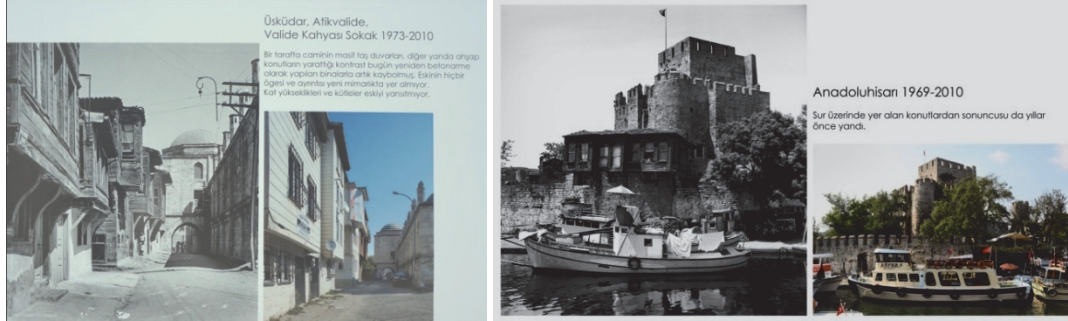
Fig. 1-2: Valide Atik Complex and its near surrounding (1973-2010), Anatolian Castle (1969-2010)
