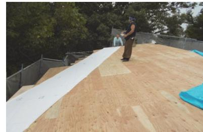
Fig. 7: Full scale drawing placed on roofboards
