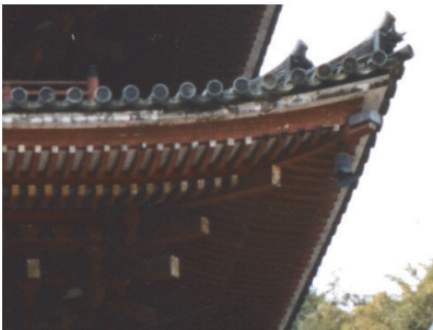
Fig. 3: Myououin, Eaves Rafters
