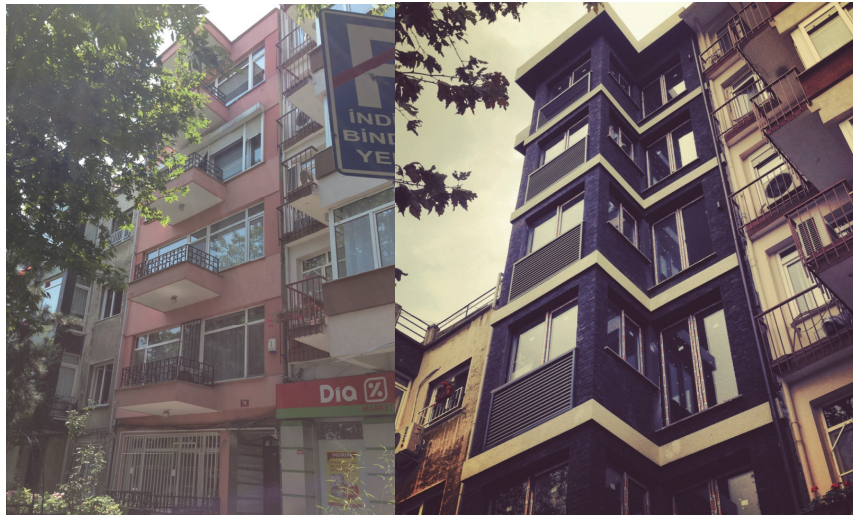
Fig. 2: Moda (A) old apartment and (B) the new one for the same plot (Architect: Hasan Alp Demir, Photographs: Serdar İncirlioğlu Archive)
