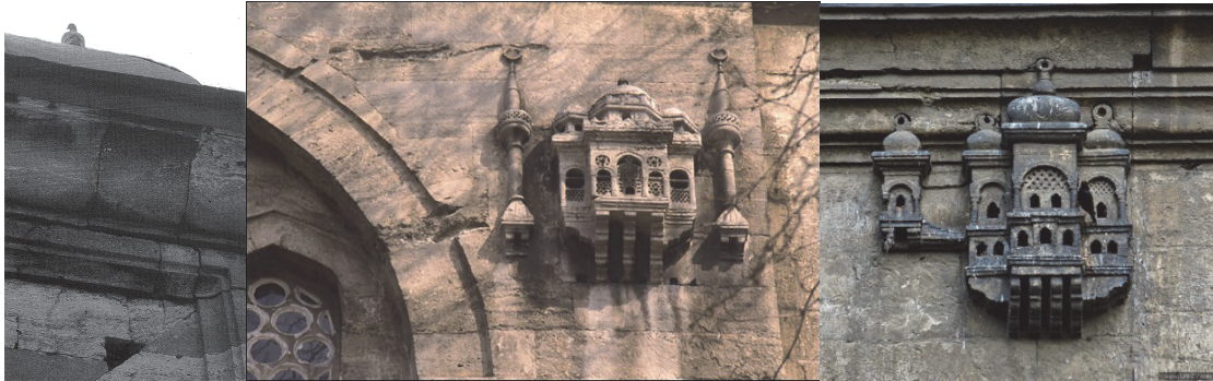
Fig. 1: On the left, an example for group one on the façade of Ayazma Mosque in Üsküdar, İstanbul, In the Middle, an example for group two on the facade of Bayezid Hasan Paşa Medresesi, İstanbul, On the right side another example for group two on the facade of Ayazma Mosque in Üsküdar, İstanbul
