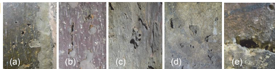
Fig. 3: Condition of the surface of the paintings (a: There are small holes and white accretions on the surface with shellac coating. b, c: The holes connect to others on the inside of the earthen plaster. d: The paint layer around the holes are disappeared in the paintings without shellac coating. e: There was an insect like to Ptinidae in the cracks on the paintings.)
