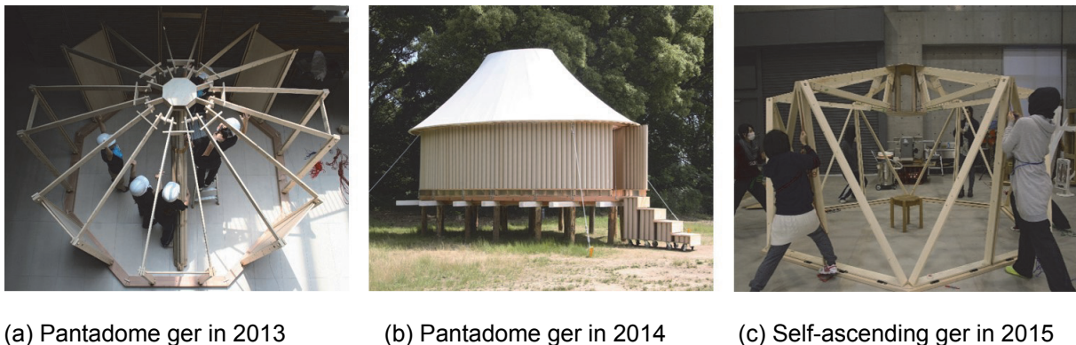
Fig. 3: Ger utilizing Pantadome, self-ascending Pantadome system
