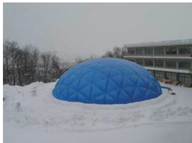
(3) 3-D air inflated formwork
