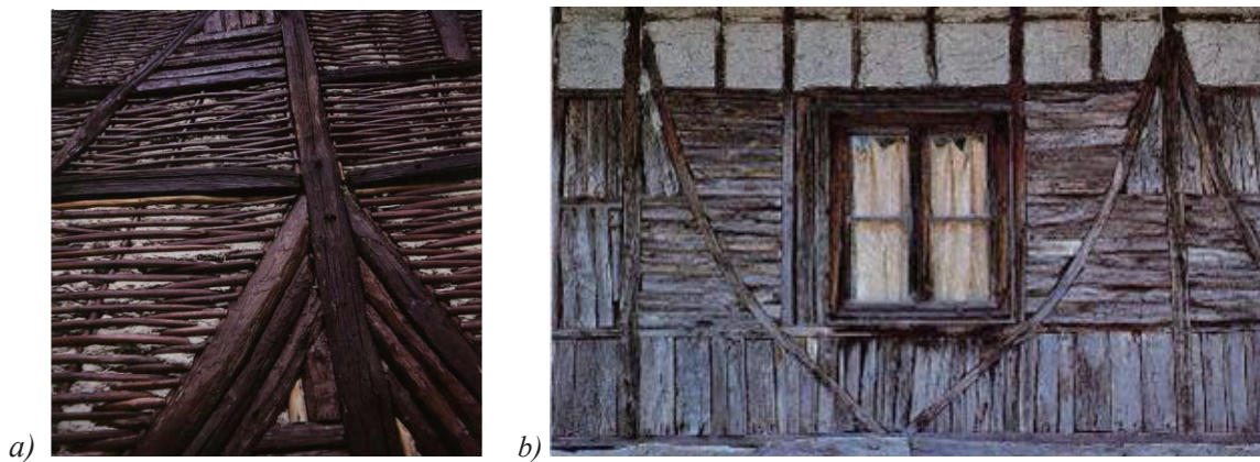
Fig. 3 Timber filled frames
