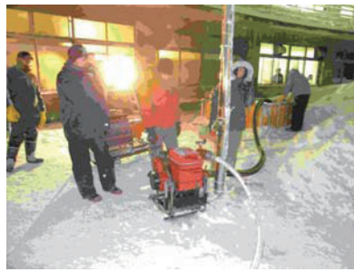
(2) Pump engine for high pressure
