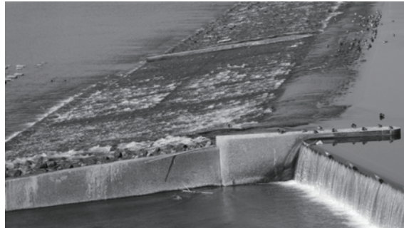
Fig. 8: Example of mechanical flushing gate (Hata-weir, the Niyodo River, Kochi)
