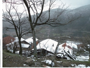
Fig. 12: Gable sides faced valley
