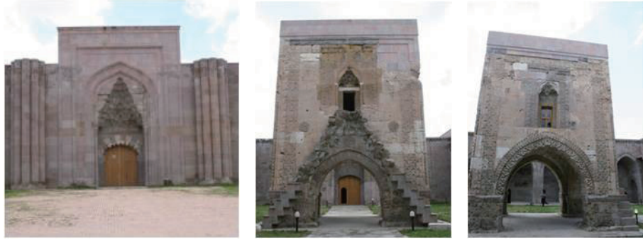
Figure.5. Photographs' after restoration
