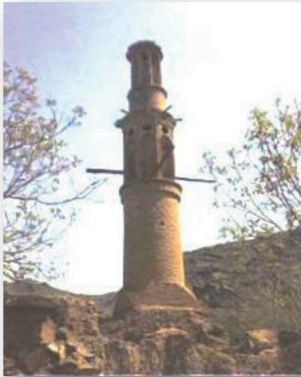
two floor deflector with circle section, Chehel Sotoon Palace, Sarhangabad village, Lorestan
