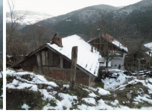
Fig. 13: Masonry walls used in downstairs
