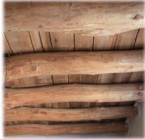
Fig. 11: Wooden boards on the beams of Ceiling
