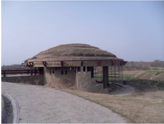
Fig. 1: (Left). Tee house under construction.
