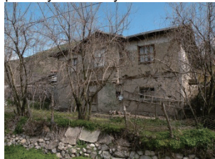
Fig. 21: House with characteristic facade
