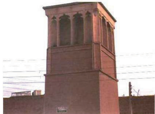
four sided deflector with square section, Kashan
