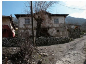
Fig. 22: House with characteristic facade
