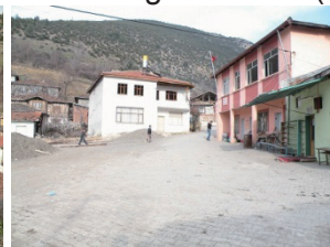
Fig. 19: Square. Village head office was in building on the right.
