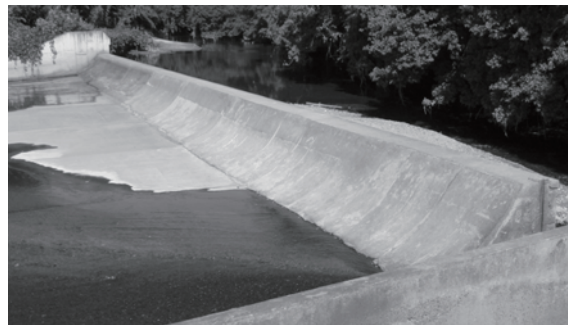
Fig. 5: Example of trapezoid shape (Kusuriya-weir, the Kuji River, Ibaraki)
