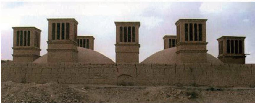
one sided deflectors- old structure of Ardakan
