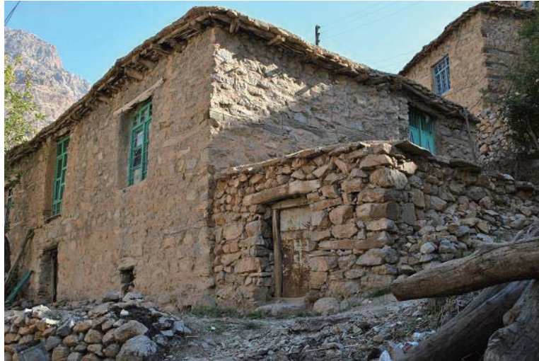
Fig. 9: (A residential block in Belbar)
