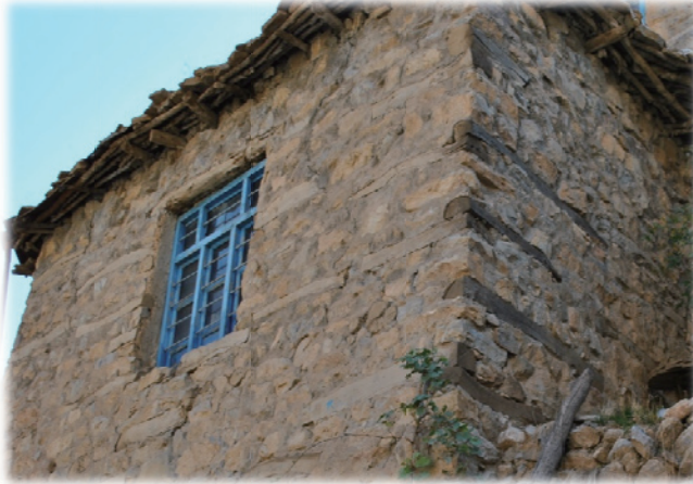
Fig. 10: Lumbers in different sections of the exterior walls (woven in corners)
