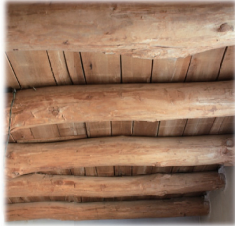
Fig. 11: Wooden boards on the beams of Ceiling
