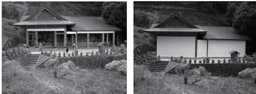
Fig. 4: The method to control a cold wind
