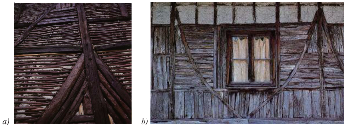
Fig. 3 Timber filled frames
