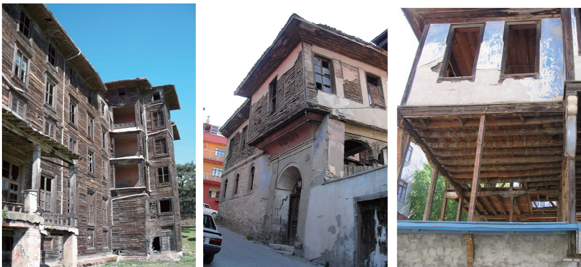
Fig. 2: Timber houses rise on foundation wall, on masonry wall and on columns
