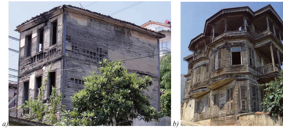
Fig. 4: Timber covered frames
