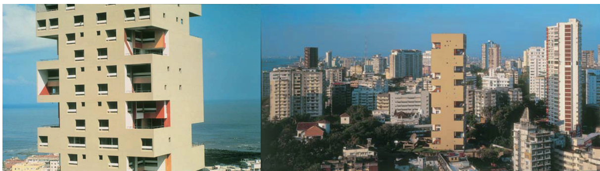
Fig. 2: Kanchanjunga Apartments in India by Charles Correa [15]
