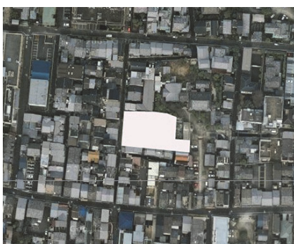
Fig. 1: aerial photo of the project site
