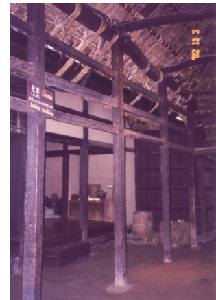
Fig. 1 Tataki floor in a traditional house
