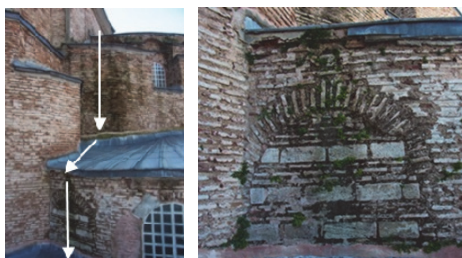
Photo 3: Trace of rainwater runoff at the outer wall of NW exedra (Location number 94)
